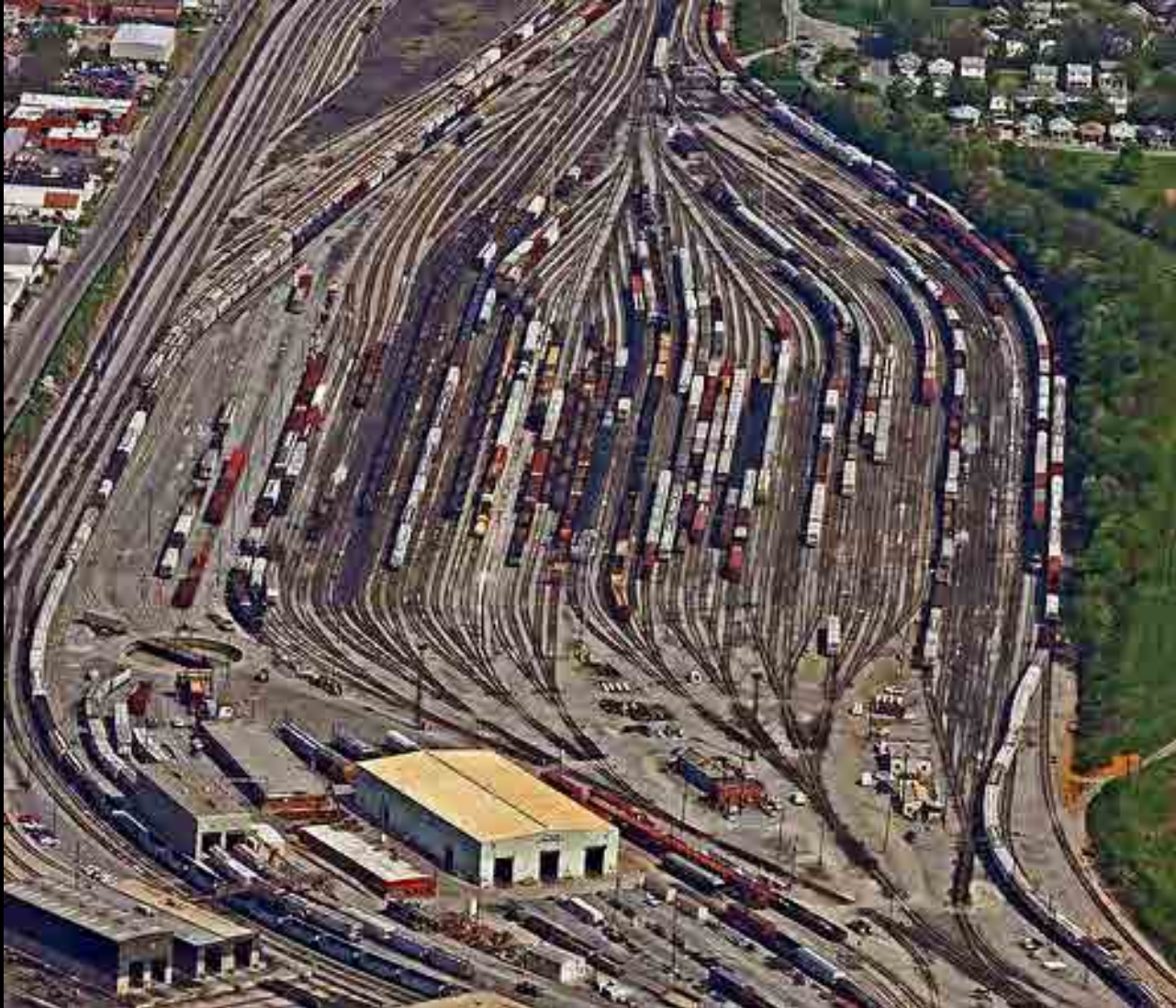
Norfolk & Southern Railway Yard – Roanoke, VA
