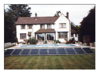
Treated timber bearers or galvanised steel bearers are laid on the earth bank to provide a fixing for the panels and to maintain an air gap between the panels and the soil. If there is no air gap then moisture in the soil could conduct heat away from the back of the panel.
