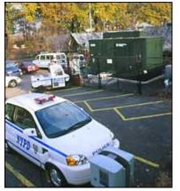
A 250-kilowatt phosphoric acid fuel cell powers a police station and electric vehicle recharging station in New York's Central Park
